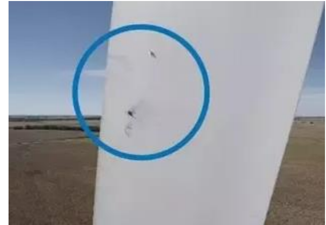
Blade cracks
