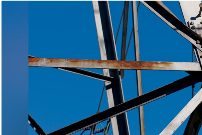
Corrosion
